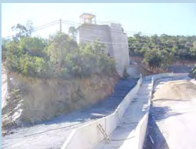
Structure for flow regulation at the Funcho side
