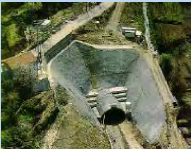
Northern Portal (Construction Phase)
