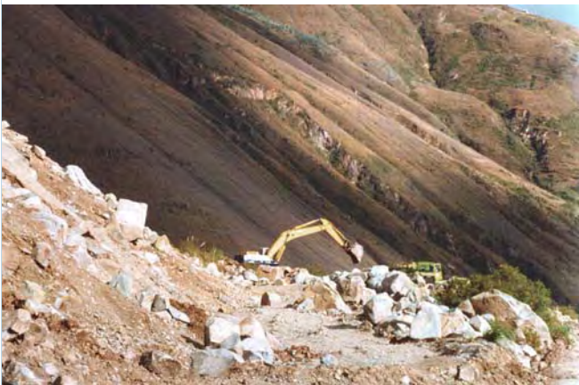
Initial phase of the slope flattening
